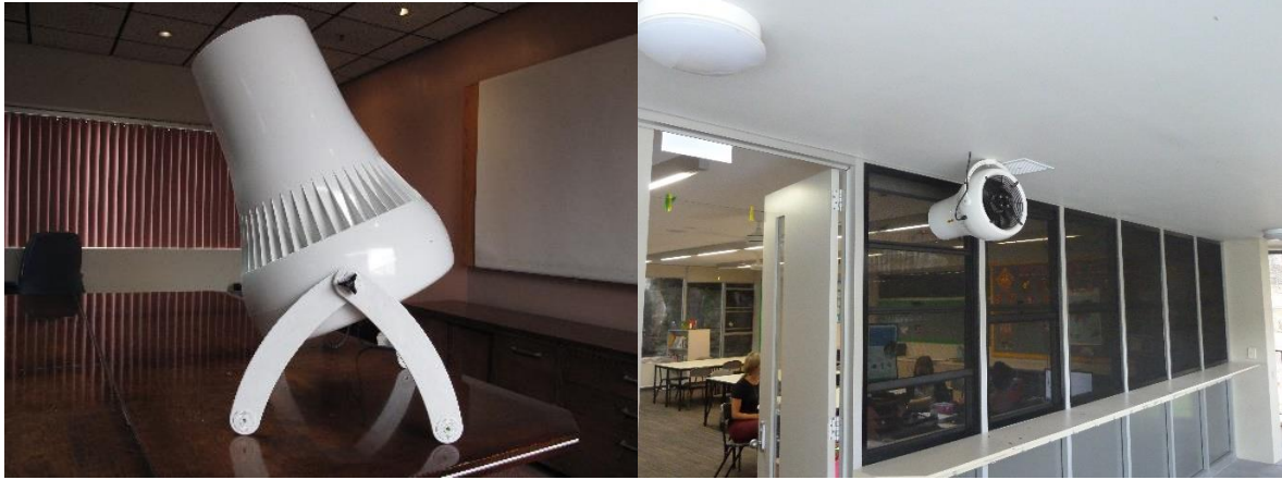
An Airius Air Pear with the Airius custom legs and one horizontally mounted in a school classroom at SCEGGS, NSW.
