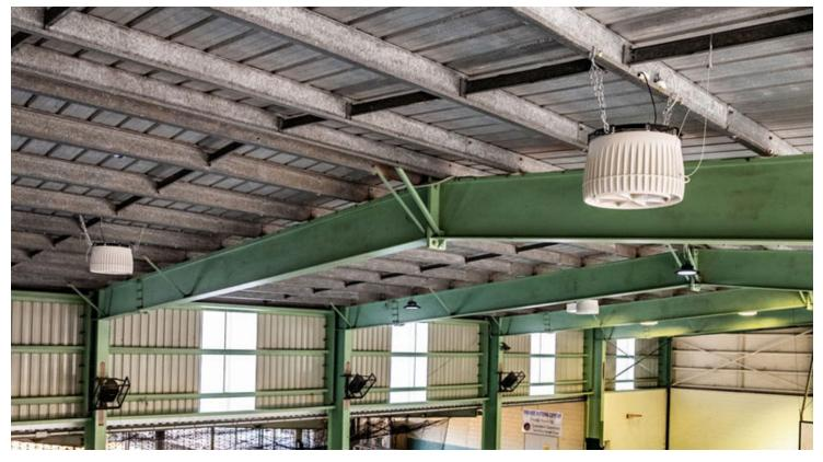
The school installed 5 x Airius G400 EC SP fans and 2 potentiometer speed controllers.
